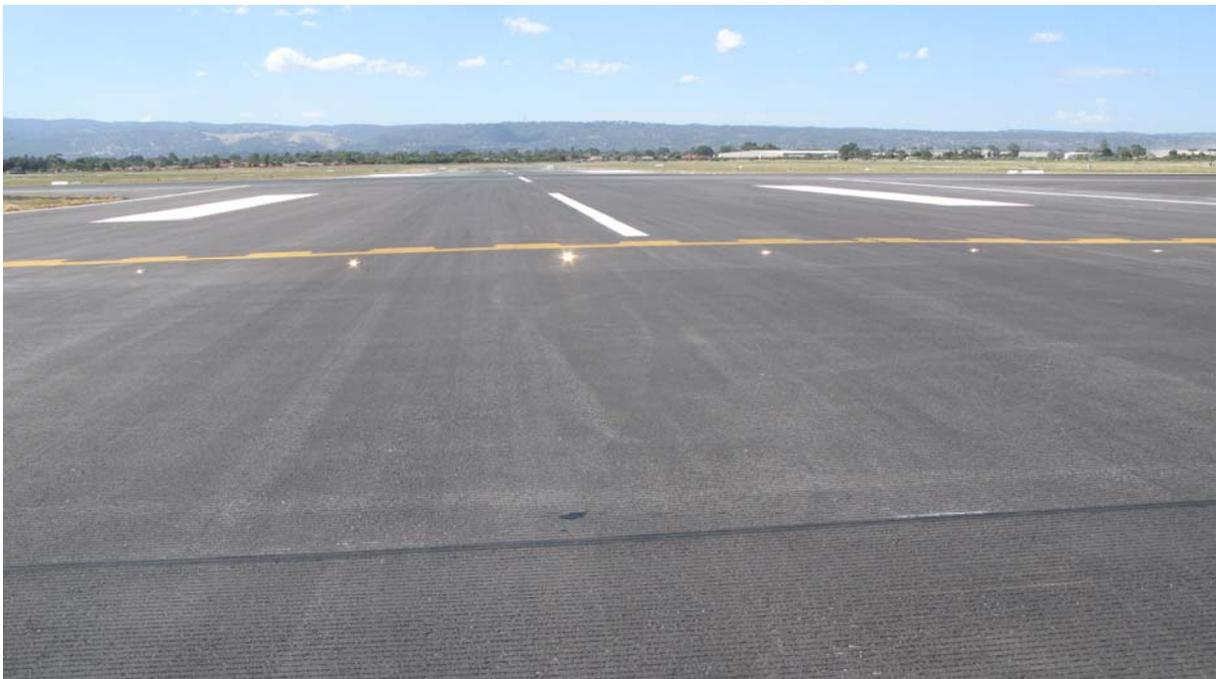
**Figure 4:** Hold Short Lights ('LAHSO Lights') are located on the runway, are white in colour and occult.
