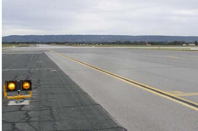
**Figure 1 left:** Holding point with yellow steady Intermediate Holding Point Lights.
